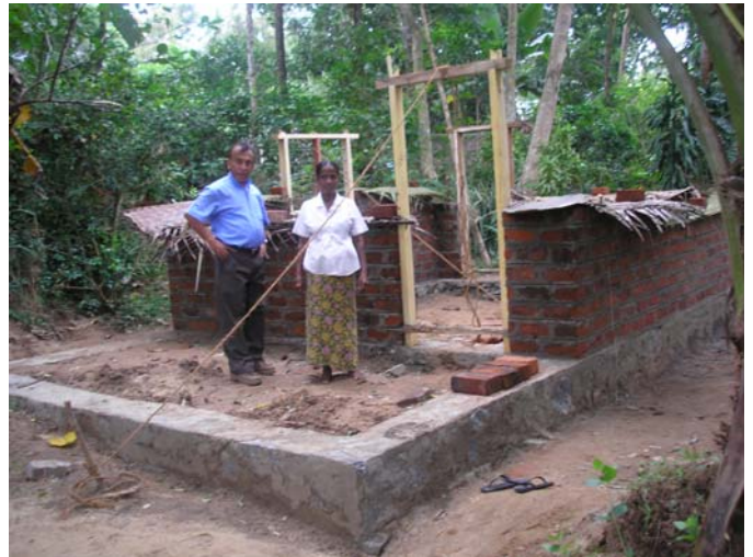
The walls of the house built up Halfway by the UCF
