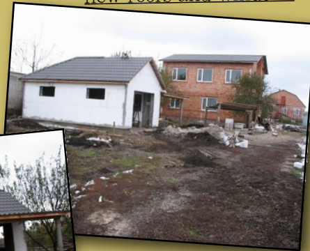
new roofs and windows
